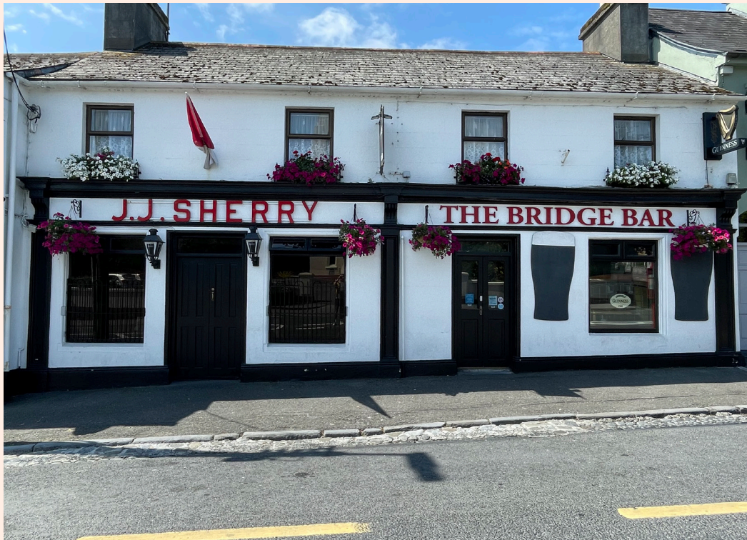
An example of a traditional sign which respects the proportion of the host building and adds to the character of the street
