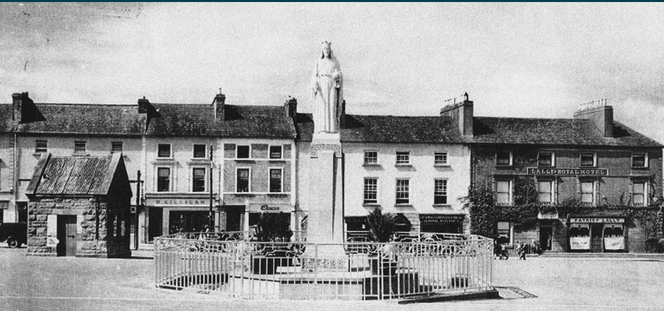
↑ Gort Inse Guaire, Co. Galway, circa 1940. The architectural backdrop to our public spaces is characterised by the disciplined rhythm of regular fenestration openings ordered along the street. This order is counterposed by the decorative shopfront which adds individuality and expresses the streets unique character. (Image courtesy of Gort Library, Cardell Collection.)
