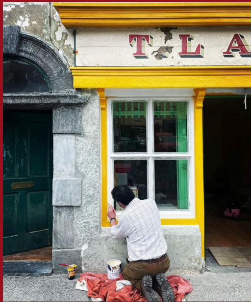
↑ The restoration of a Georgian style shopfront in Gort Co. Galway is an excellent example of both well selected colour scheme and hand painted signage.
